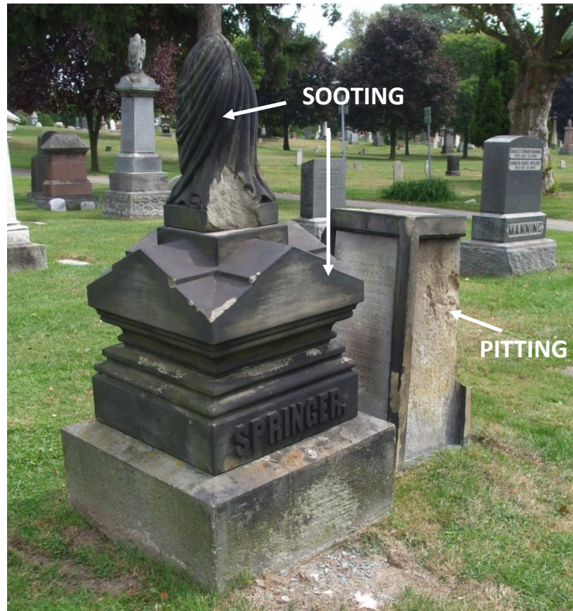
Figure 5.5 Monument exhibiting both sooting, particularly on the upper extremities, and pitting, which has affected one of the two visible panels of lettering. The monument also toppled during the summer of 2010 (Fall 2010).
