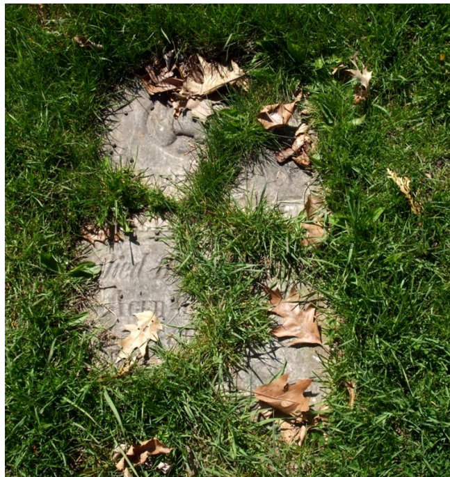
Figure 5.7 Marble slab monument that has cracked into four pieces and is now laid flat.
