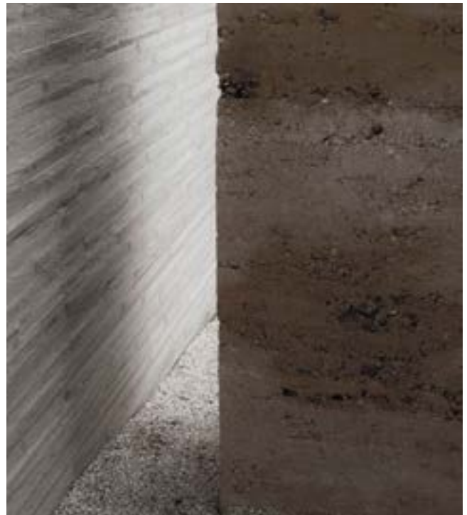
Fig. 7.34: use of rammed concrete at Kolumba Museum courtyard in Cologne by Vogt landscape architects; source: Danish Architecture Center, 2021
